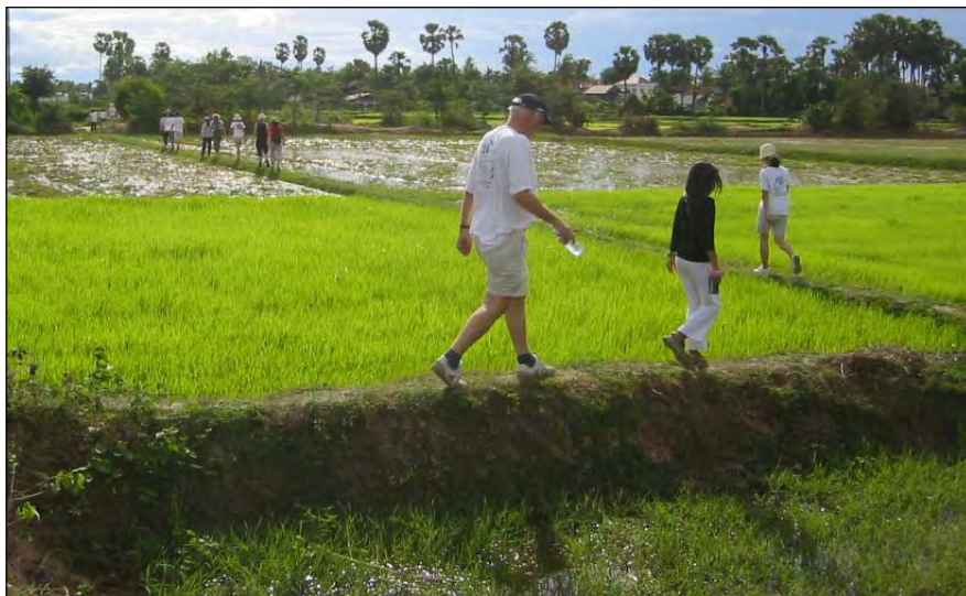
Figure 7.4: Typical earth embankments associated with rain fed rice
