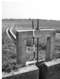
Tertiary canal and Gate
