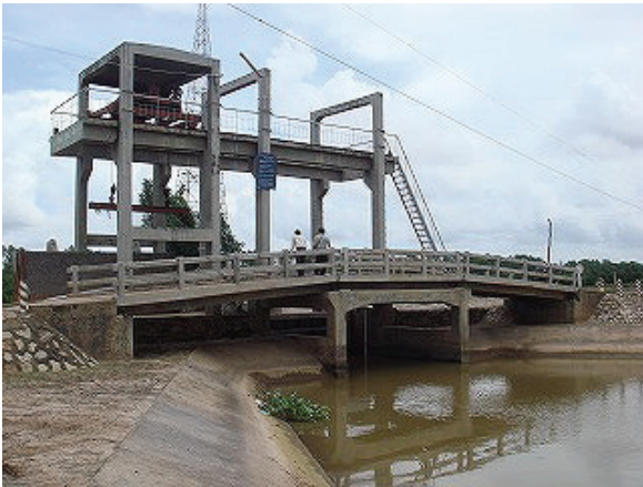
Sluice at Long Hai station
