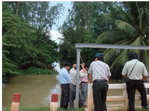
Observing HL 6 sluice
