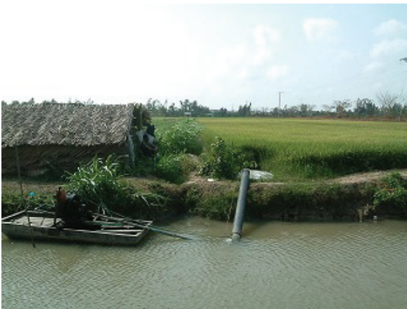
Water delivered by individual pump
