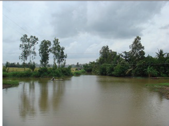
Long Hai sluice in side command area
