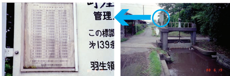
Figure 3.3 Bulletin board informing water users in each sub-irrigation system of the water delivery rotation at irrigation turnouts
