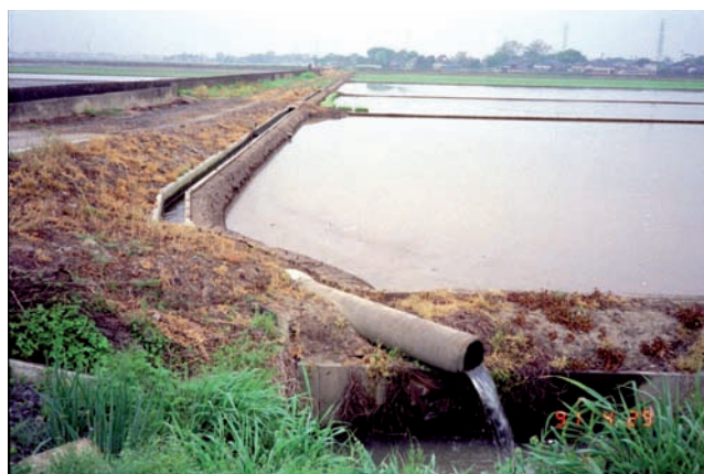
Figure 3.8 Overflow from a tertiary canal
