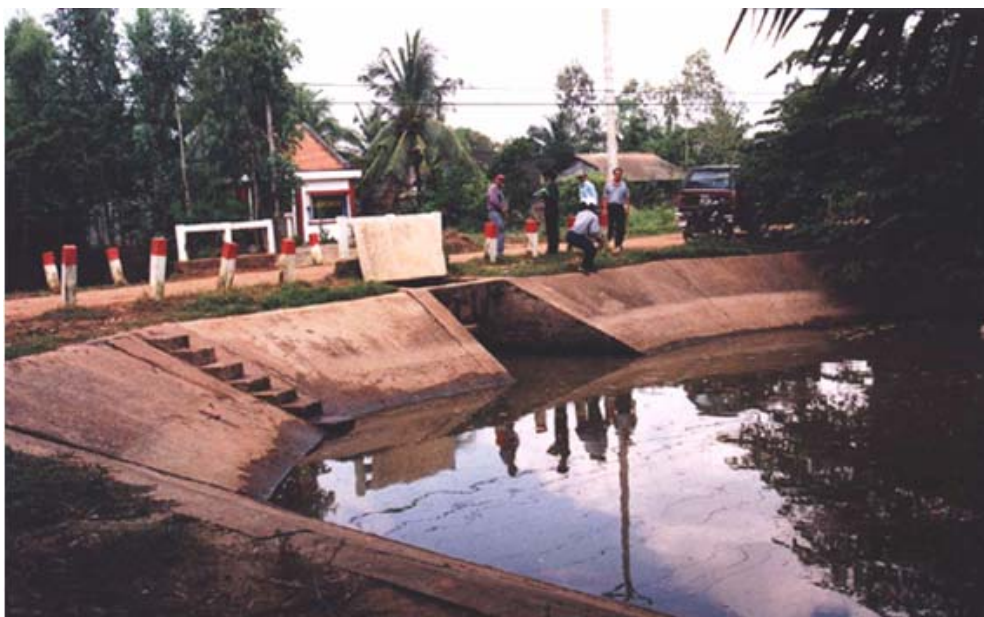
Photo 1: A photo of HL6 sluice
