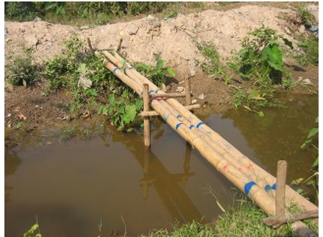
Construction of Bamboo Bridge for all Measurement Points
