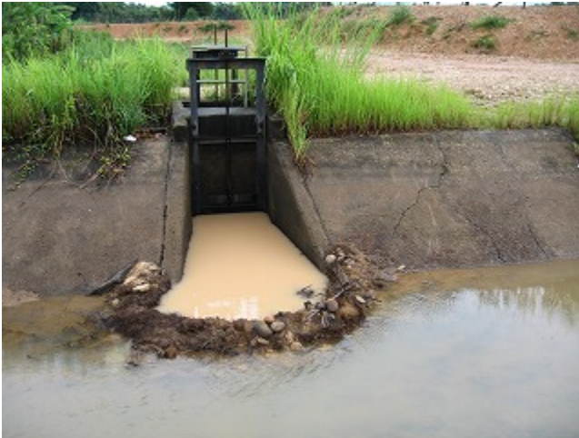
Secondary Canal Intake
