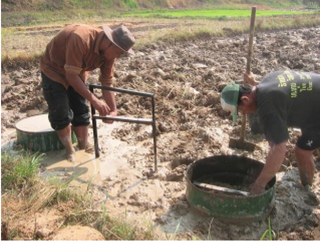
Installation of ETc and Percolation Measurement
