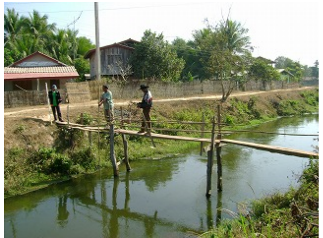
Flow Measurement Conducted at Main Canal
