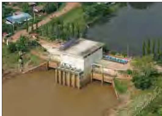
Plate 16. This watergate across the Huai Mong, a Thai Mekong tributary, prevents rising Mekong floodwaters from running into this tributary, and also blocks migrating fish and fish fry from accessing the tributary and flooded areas. Similar effects would be expected if the lower Songkhram River were to be dammed.
