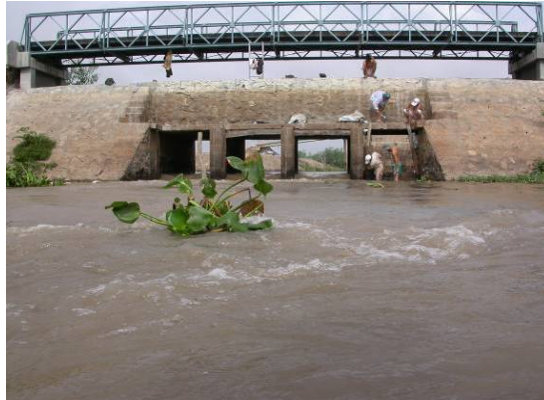
Figure 3 Example of a culvert with a number of openings.
