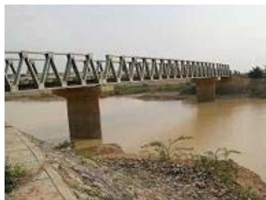
Figure 5.16 Bridge as through-flow structure.
