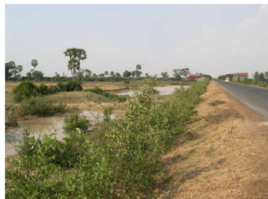
Figure 5.5 NR11 at the spillway.
