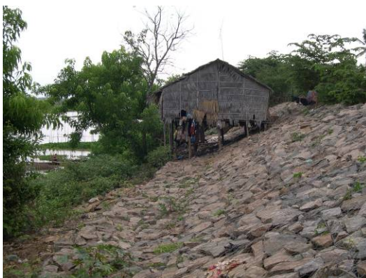
Figure 5.4 NR11 section with slope protection (rock filled gabion mattresses).
