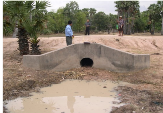
Figure 5 Example of a small culvert.
