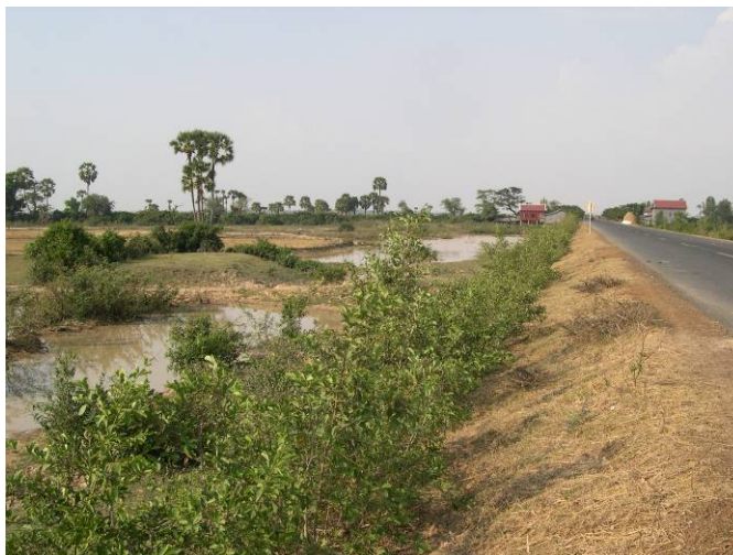
Figure 9 Vegetation to protect a slope against wind waves.
