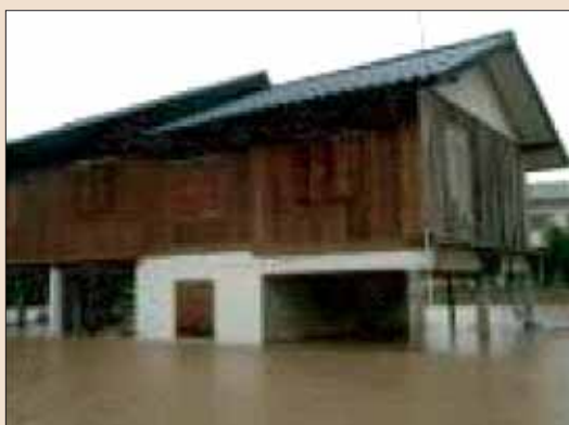
Flash flood damage in Chiang Rai, Thailand
