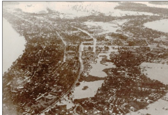
Figure 5.6 The extent of flooding across Vientiane on the 1st September 1966, indicating the potential disaster that was averted by the prompt actions taken during mid August, 2008.
