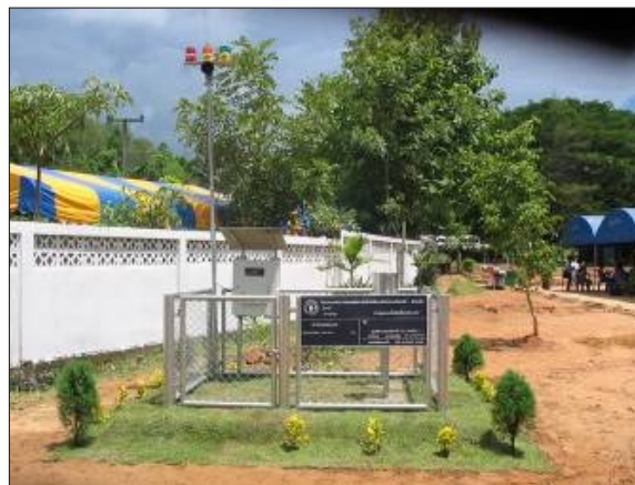
Figure 6.10 A component of the flash flood and landslide monitoring network.
