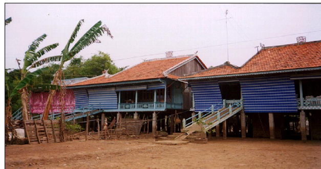
Figure 6.12 Structural flood mitigation measures implemented in the delta—schools and houses raised on piles.
