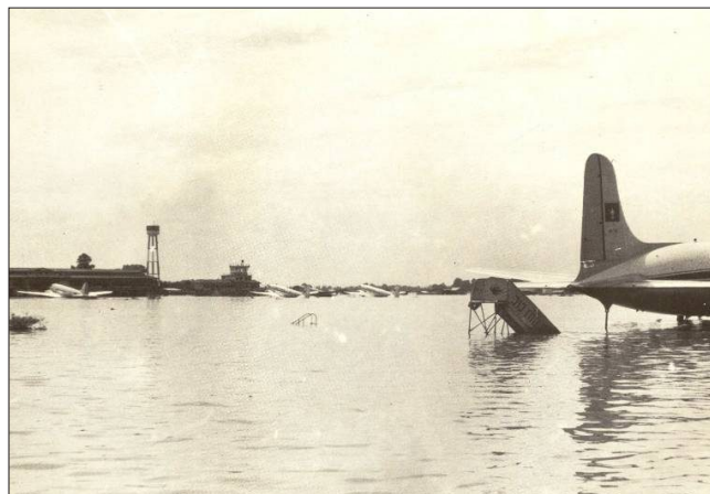
The flooded runway at Wattay Airport.
