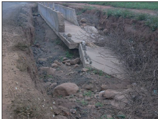
Figure 42. Destroyed irrigation canal in Dak Lak as a result of Typhoon No. 2 and a flooded village in the Se San Basin following Typhoon No. 5.
