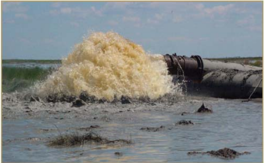
Dredged sediments being placed in open water to restore marsh that has been lost.
