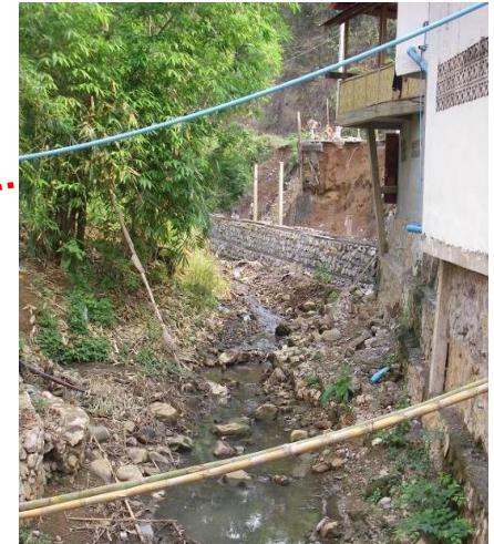
Corridor of residential blocks along the Houay Xon
