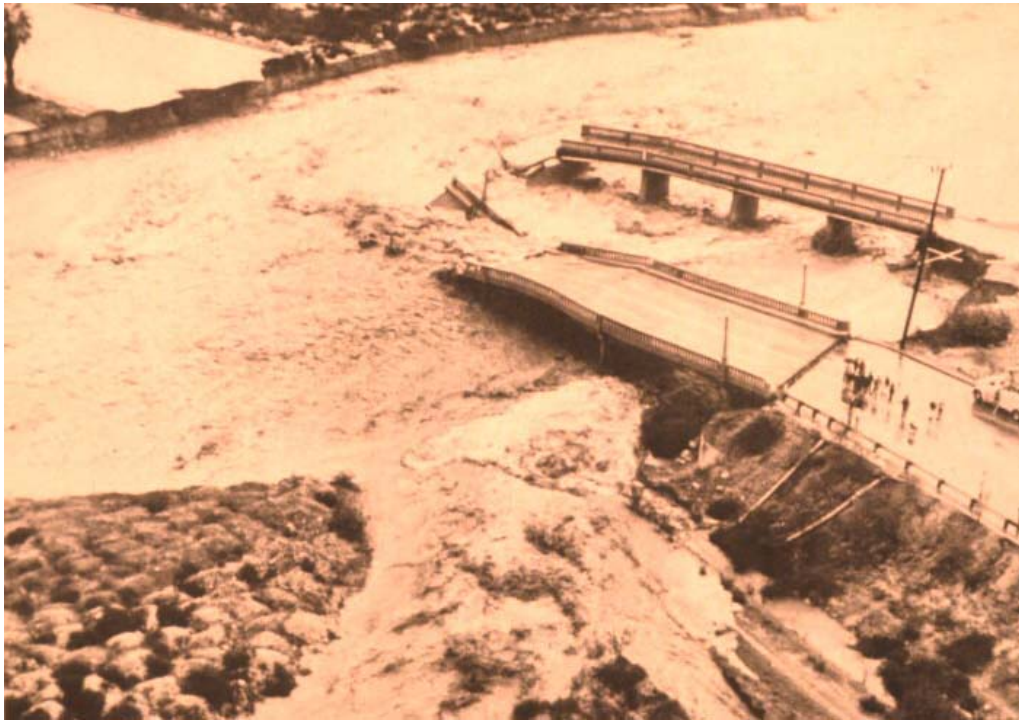
Tujunga Wash, Los Angeles washing out the Foothill Blvd bridge in 1969
