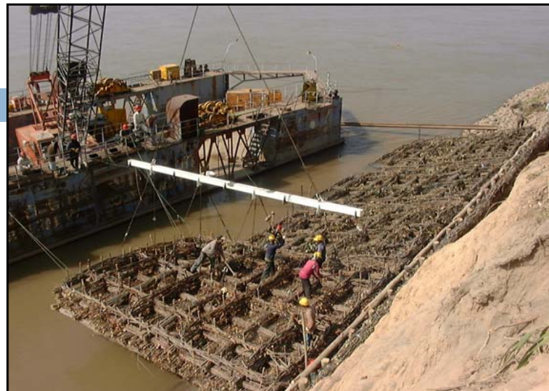
Installing foot protection Soda mattress
