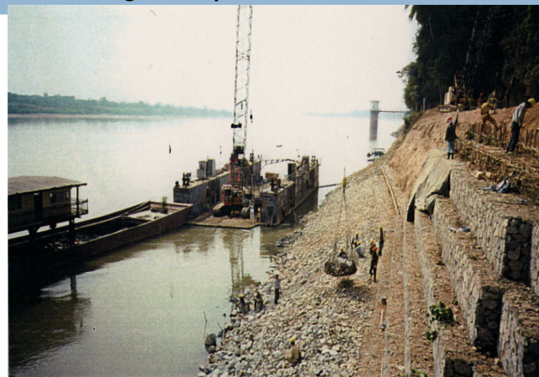
Placement Rip rapping on Soda mattress
