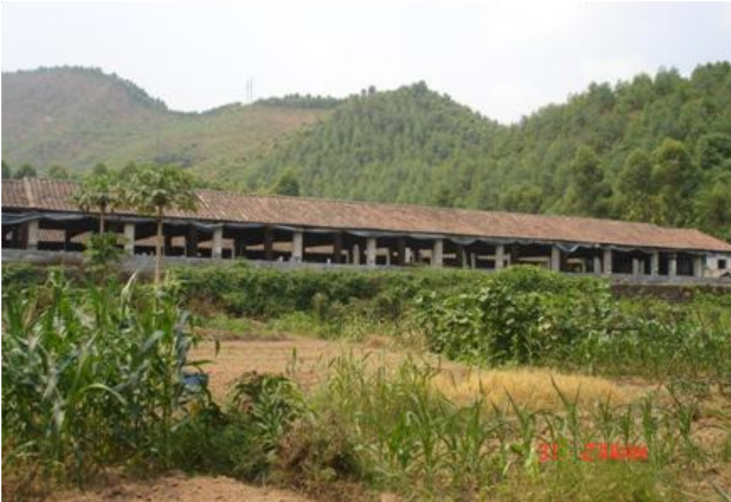
Figure 2.4c Contemporary pig wastewater treatment system of Louxing Pig Farm in Bolou County(博羅縣), Guangdong Province(廣東省), China
