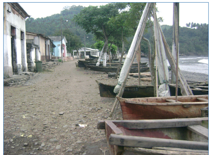
Beach erosion and boats on the street
