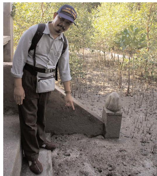
Figure 5: Wat Khun Samutchin. Three steps are buried below the present ground level. Photograph taken by Ms Vareerat Unwerawattana on 24 May 2007. Location is shown in Figure 2.
