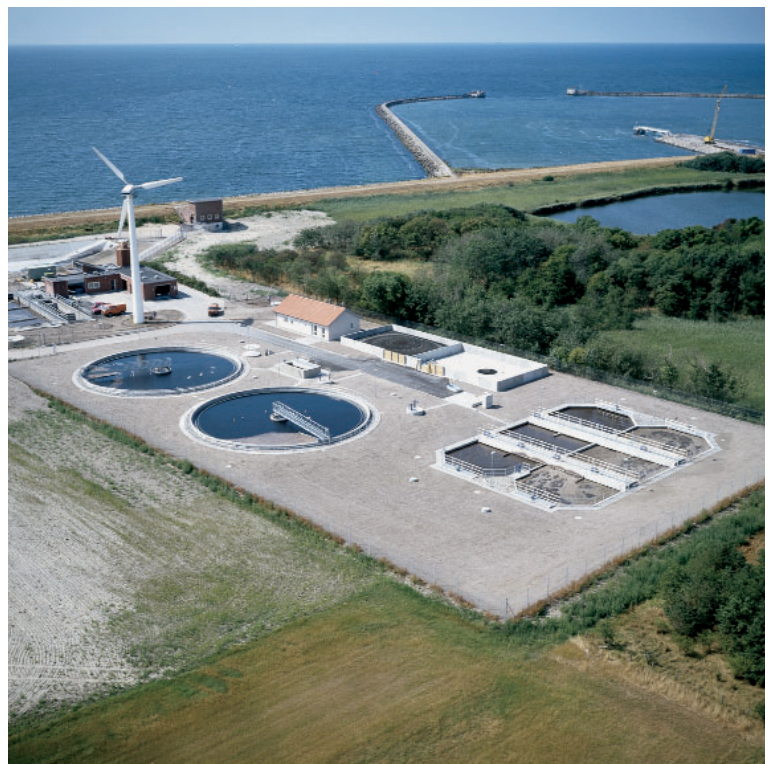
Waste water treatment plant at Rødbyhavn, Denmark. Photo: Biofoto/Mr. Lars Havn Eriksen, 1994.
