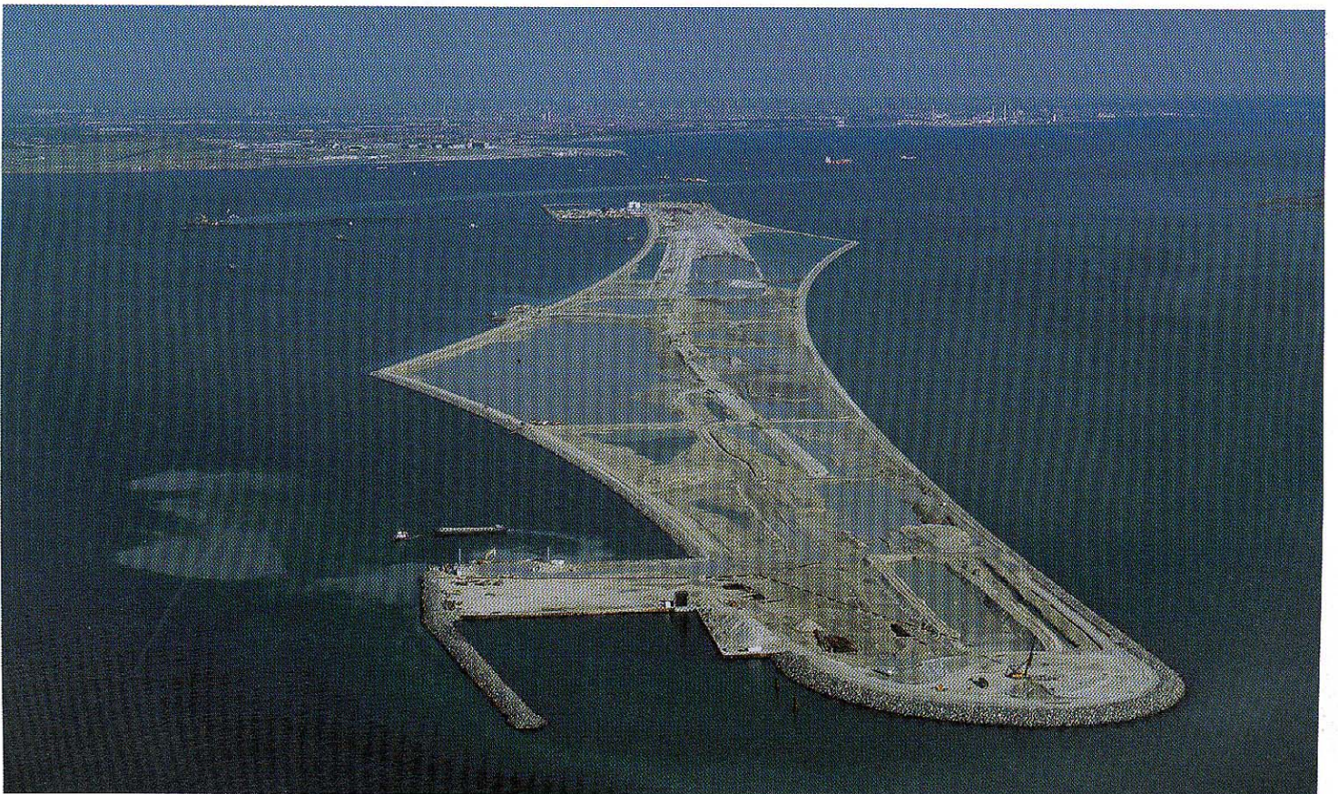
Figure 5: Use of marine sediments: Construction works. Construction of an artificial island for the fixed link between Denmark and Sweden (Photograph courtesy of Øresundskonsortiet).
