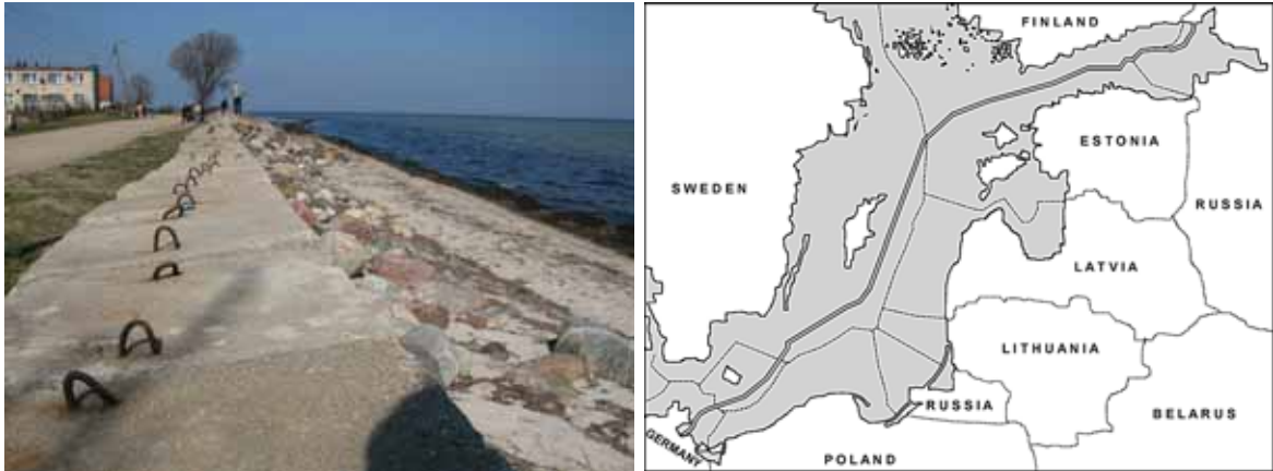
Figure 6.3.3. Left: concrete-stone coastal protection on some parts of the Hel Peninsula in Poland. Right: planned route of the Nord Stream pipeline ( www.nord-stream.com ).
