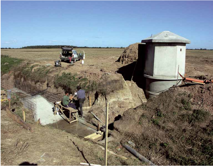
The Graisupis stream monitoring post under construction in Lithuania
