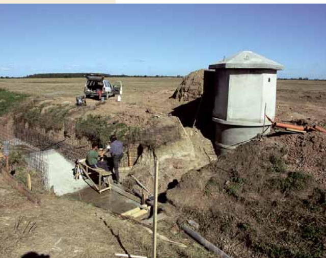
The Graispis stream monitoring post under construction in Lithuania
