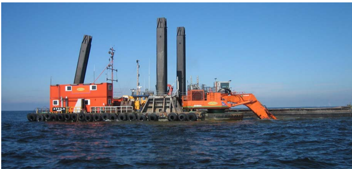
Dredging of a ship lane. Photo: Metsähallitus 2007
