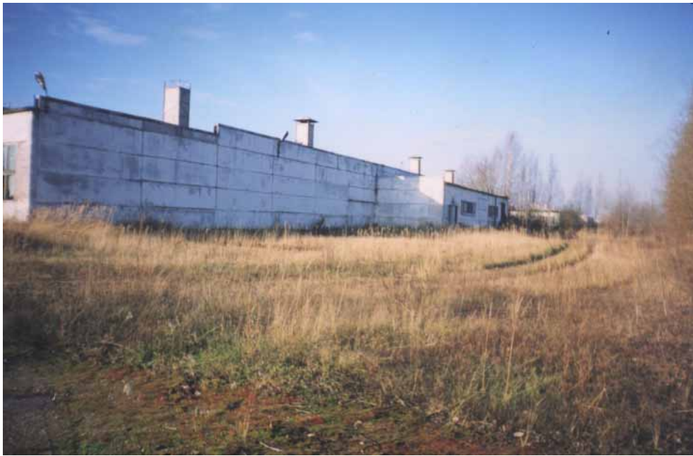
Figure 14. Sputnik Complex. Third production line.
