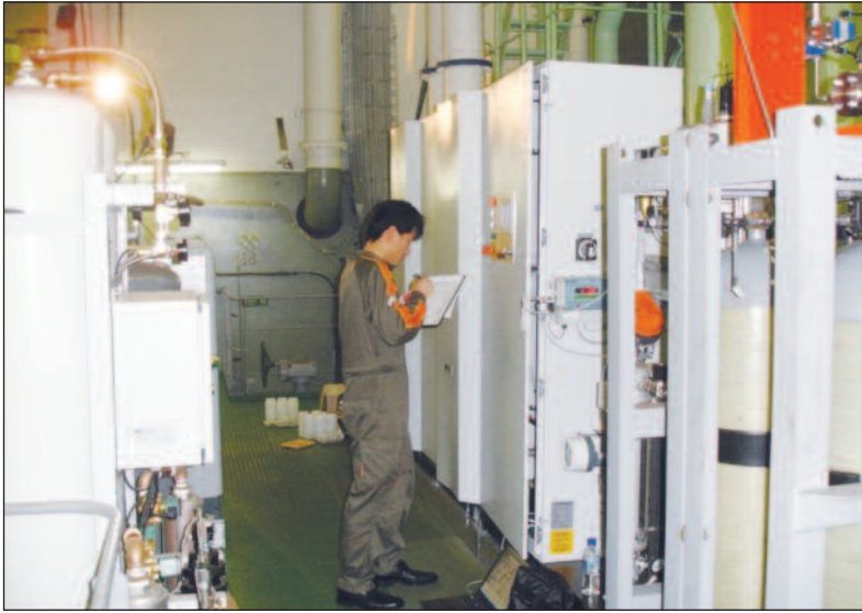
Figure 11. NK-O3 system fitted on the container ship M.V. Hyundai Hong Kong.
