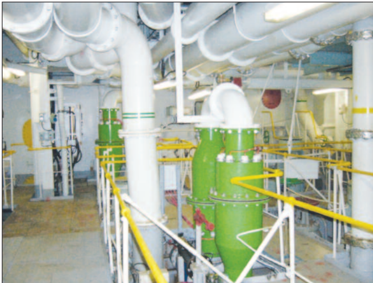
Figure 1. UBWT system installed on MV “Toronto” (Source-Wilhelmsen Group)
