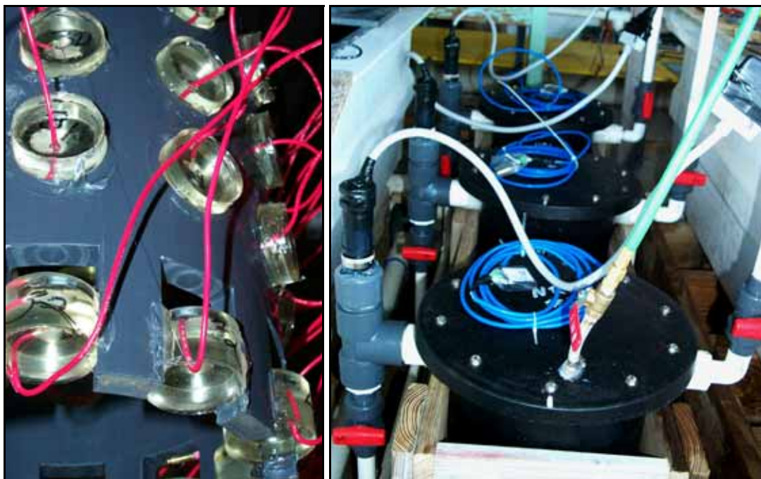
Figure 2. Experimental setup to examine rates and mechanism of corrosion under the deoxygenated conditions produced by the Venturi Oxygen Stripping™ system.
