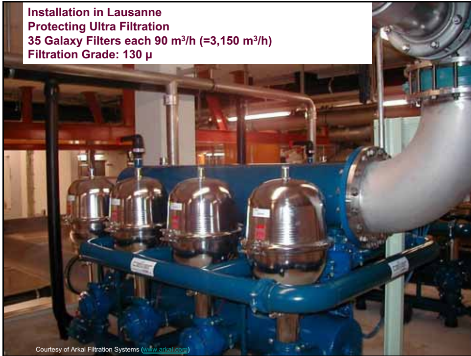
Figure 4. Ganging together of modular disk filters.
