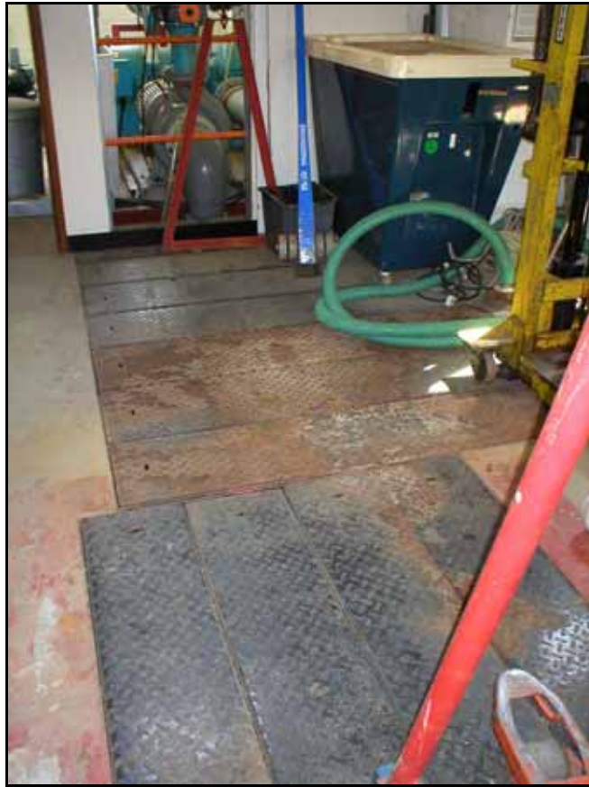
Figure 1. Top of water tanks with access hatches.
