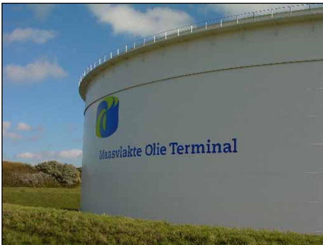
Figure 2. Maasvlakte Olie Terminal, Rotterdam.
