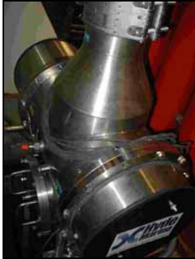
Figure 8. Aquionics UV Chamber, Coral Princess.
