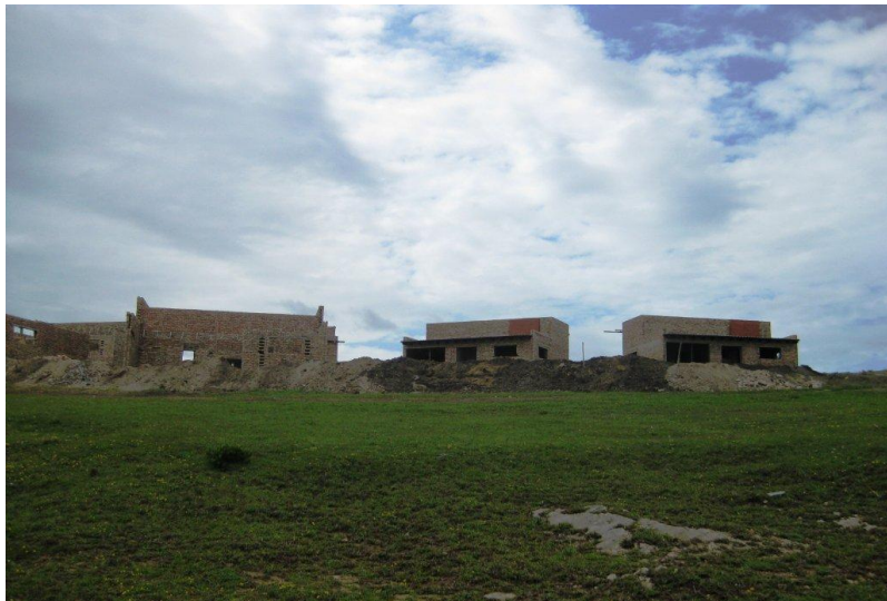
Figure 8: The ASPIRE Art Colony under construction in Hamburg in December 2010.
