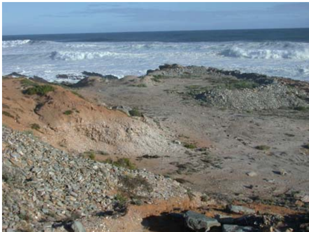
Plate 17. An extreme example of oversized dumping around the classifier site above the high water mark.
